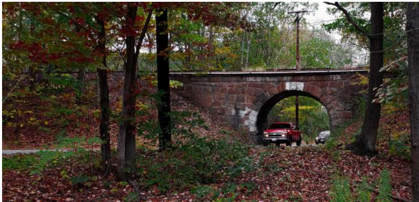
Figure No. 16: Picture of a Stone Arch Bridge by Riverside Park
